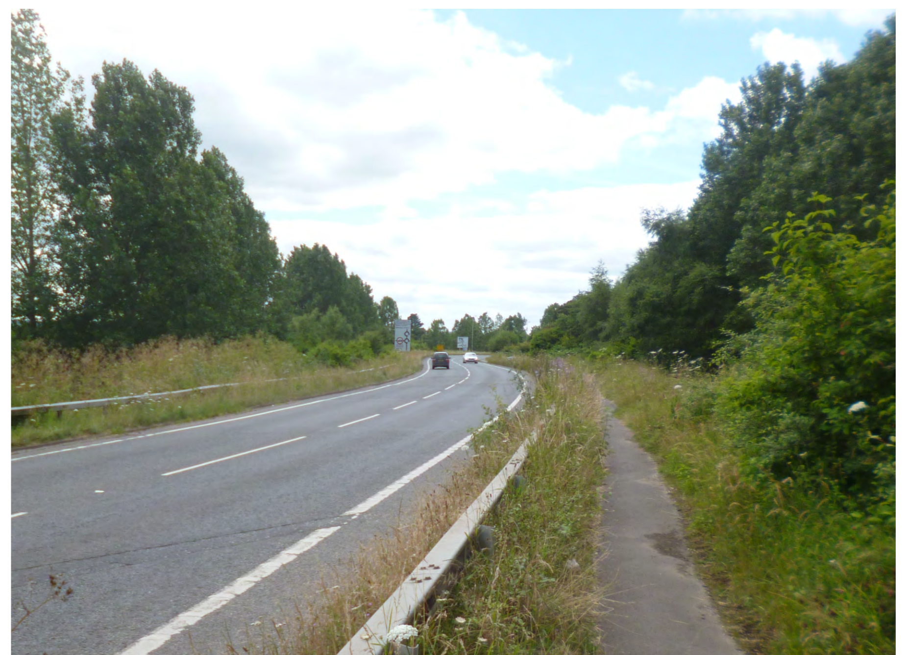
Nosworthy Way looking west towards roundabout
